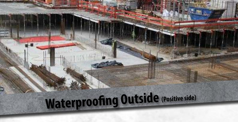
Positive side waterproofing means sealing on the water-facing side. That means outside sealing, for example basements, underground garages or tunnels. Depending on the building situation and requirements, various product systems are available.
