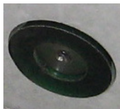
Good fixed on the formwork
