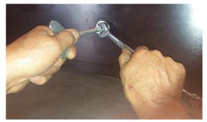
The BH-Tubeholder is well set for the Corrugated steel tube if it can be slide easily and without resistance into the steel corrugated tube. After tightening the BH-Tubeholder with the corrugated steel tube to the formwork. The correct setting can be checked because the steel pipe can no longer move or rotate manually.
