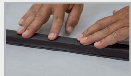
Press the swelling tape into the adhesive bed
