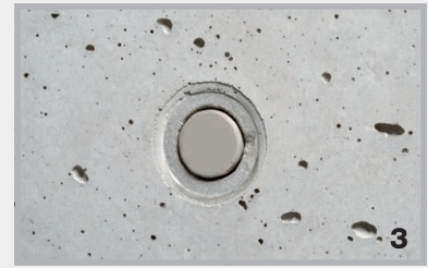
Flush seal for distance tubes with lip.
