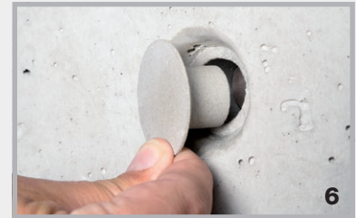
After inserting the STOPPER in, a cone can be glued in.
