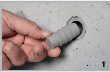
The STOPPER in is pushed into the distance tube.
