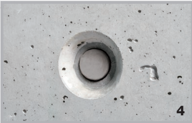
Flush seal for distance tubes with cone.
