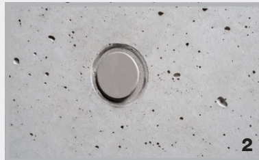
Sealing of distance tube with lip
