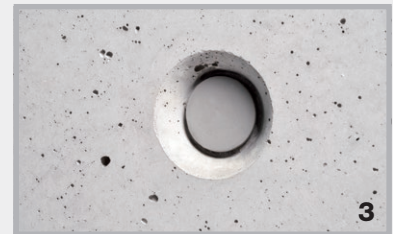
Sealing of distance tube with cone
