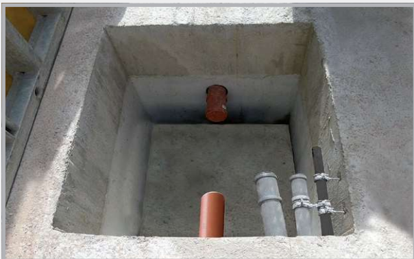
Following concreting: illustration shows the pump sump (light grey) and concreted foundation (dark grey).
