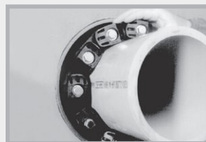
Push MASTER-SEAL into the annular gap
