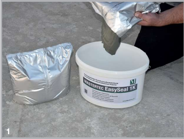
1 Open the bags and pour the coating into the bucket.
