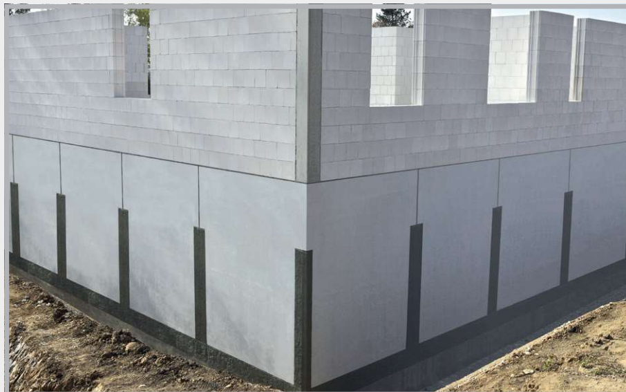
Sealed horizontal and vertical joints
