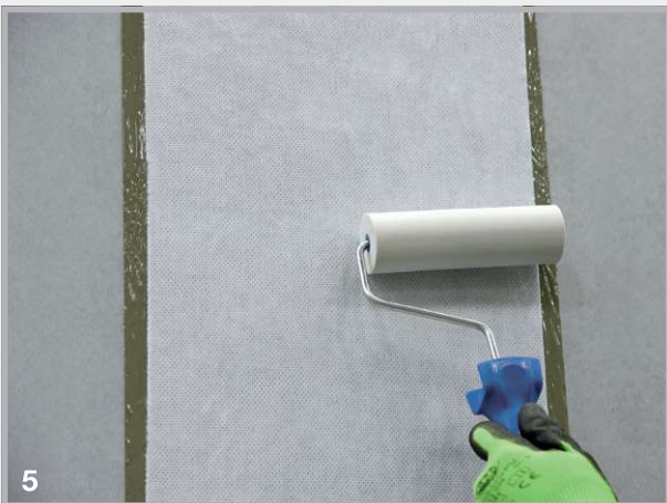
5 Roll the non-woven into the coating completely with the pressure roller. This working step makes it possible to apply the second layer after approximately 2-3 hours, depending on the temperature and air humidity.
