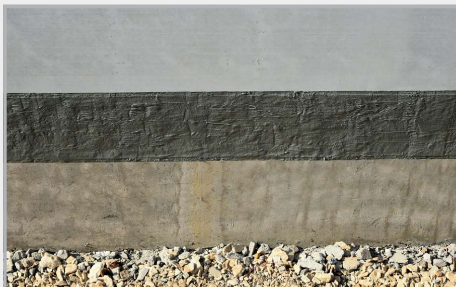
Sealed horizontal joint
