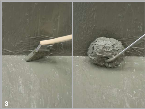
3 There is a brush and corner roller for the fillet and other areas.
