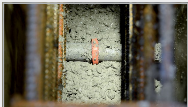
At the construction site
