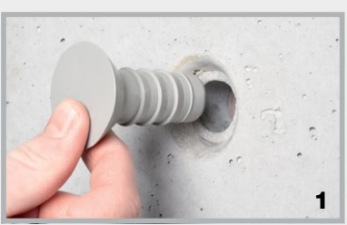
1 Push the STOPPER maxi into the distance tube
