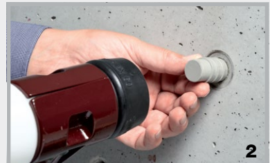
2 The STOPPER in is driven in with a 1500-2000 g hard rubber mallet.
