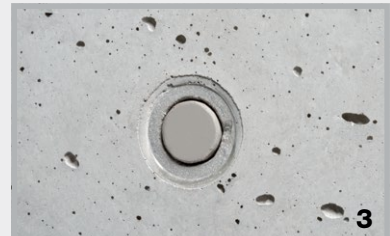
3 Flush seal for distance tubes with lip seal.
