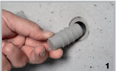
1 The STOPPER in is pushed into the distance tube.
