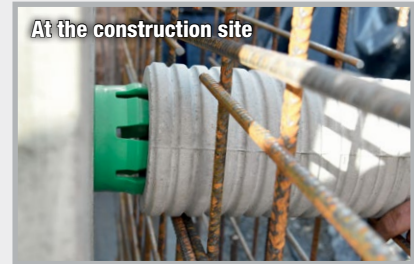
Fastening without screw adapter with nails. For easy stripping of formwork, do not use screws.
