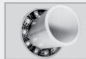
MASTER-SEAL installation complete
