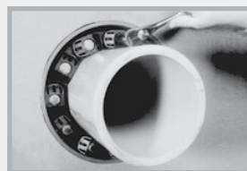
Tighten each screw one by one in a circular direction by turning once until all modules are evenly tightened
