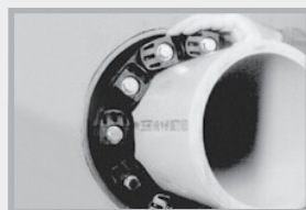
Push MASTER-SEAL into the annular gap
